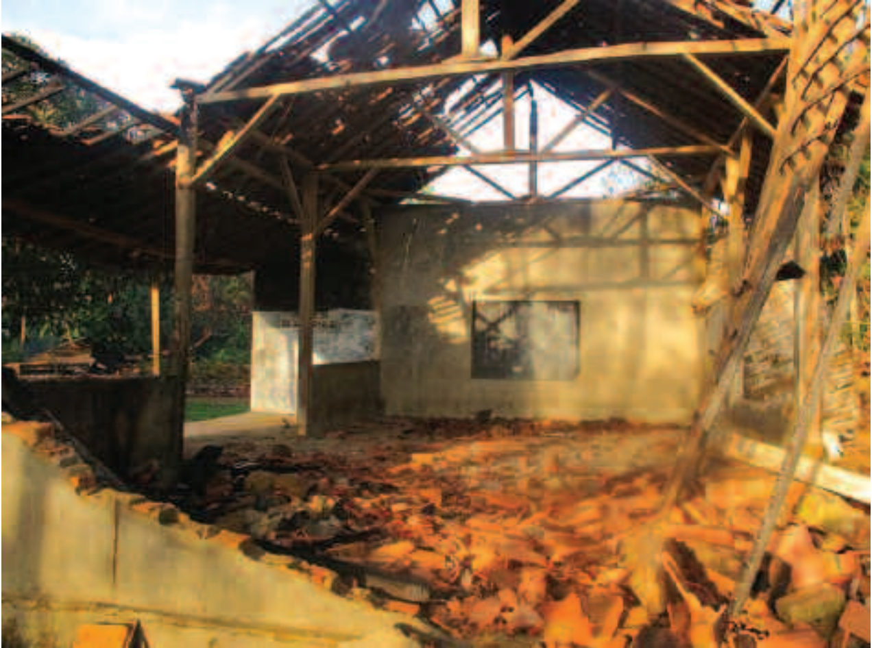
The ruins of a Shia school that was set alight when hundreds of Sunni militants attacked the Nangkernang hamlet in Sampang regency, Madura Island, Indonesia on 29 December 2011.
