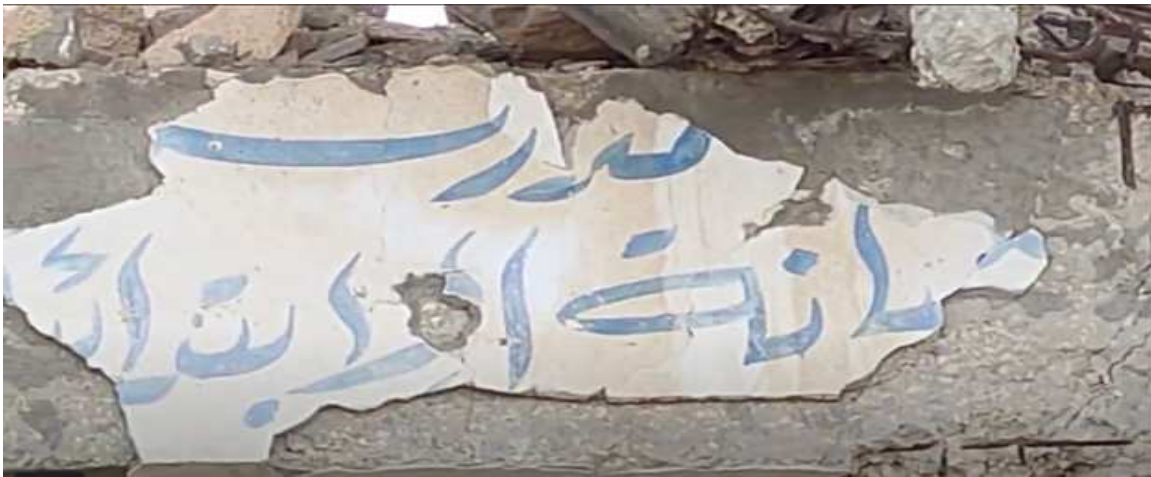
Image 2: Part of the primary school sign can be seen on the side of the destroyed building.
