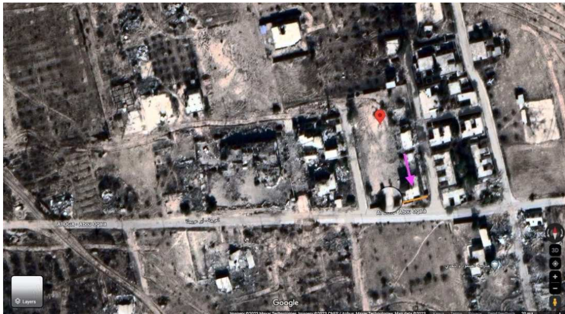
Image 5: Satellite shot showing the actual dilapidated building, the southern wall, and a small building on the edge of the school.
