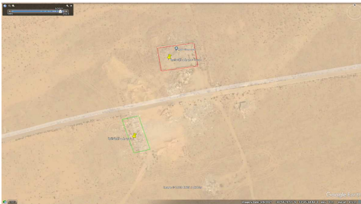
Image30: A satellite image of the two schools in March 2021 shows the two schools and some of the village buildings after the destruction, the Primary School in the green rectangle, the Preparatory School in the red rectangle.
